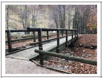
To overcome rough stretches represented by stream beds, which run through the valley, two wooden crossings were built with relative support and protection fences.
