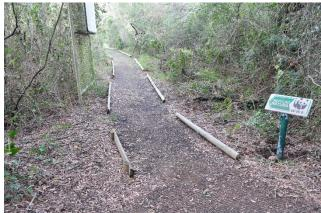
The path is one meter wide and is bordered on both sides, along its entire length, by two wooden curbs that make the route visible and safe; The guides were made with treated fir strips and fixed to the ground with wooden pegs.
